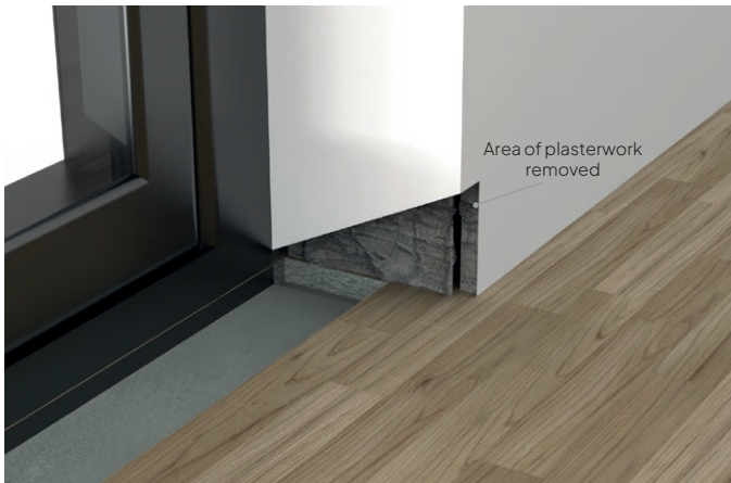
Relieve the plasterwork, allow enough room for the tectite to fit flush to the wall.
